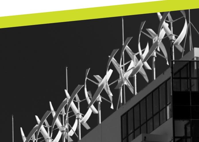
Small scale building integrated wind turbines need to have access to laminar wind (uninterrupted flows of wind in parallel layers), however many areas in larger CBDs will have quite turbulent wind flows and therefore be unsuitable.
